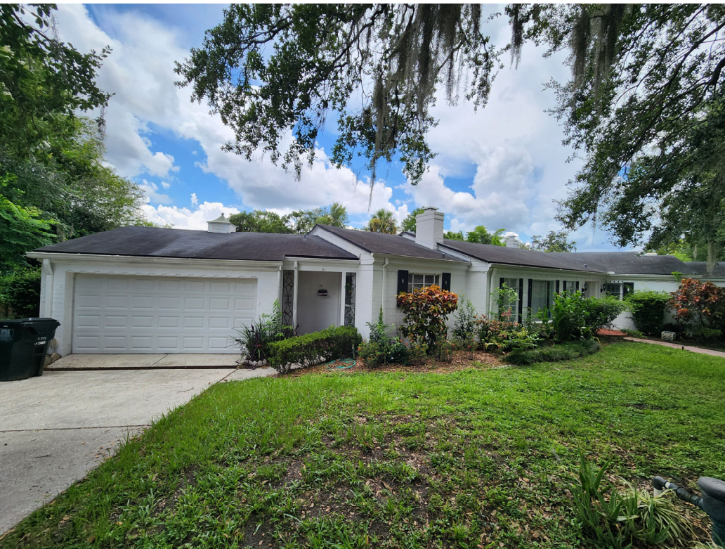
Looking at garage from driveway
