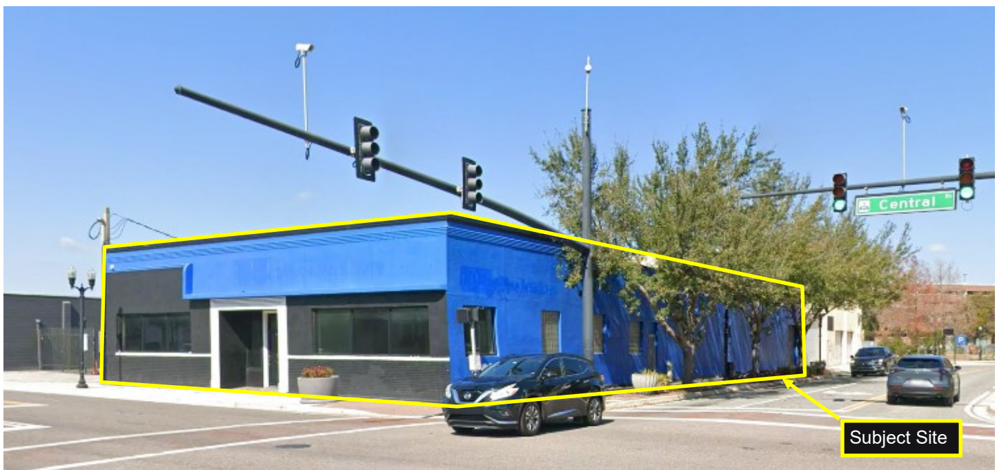
Pictured above: View of subject site from intersection of Central Blvd and N Division Ave, showing building façade and landscaping.
