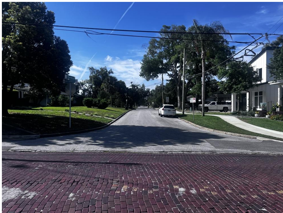
View south of Thornton Ave from Lake Highland Dr
