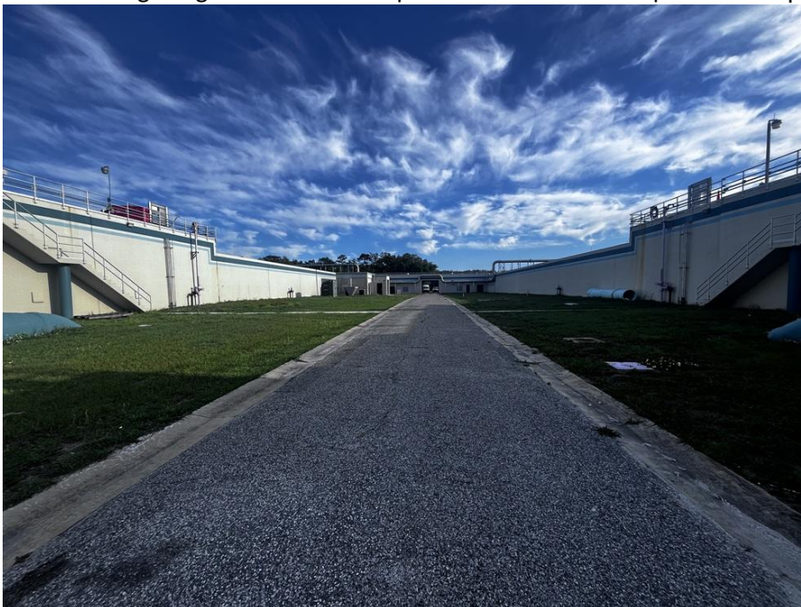
View north of Iron Bridge Regional WRF Bardenpho Blower Electrical Improvements project area.
