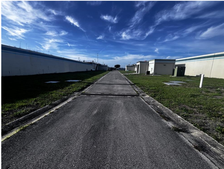
View south of Iron Bridge Regional WRF Bardenpho Blower Electrical Improvements project area.
