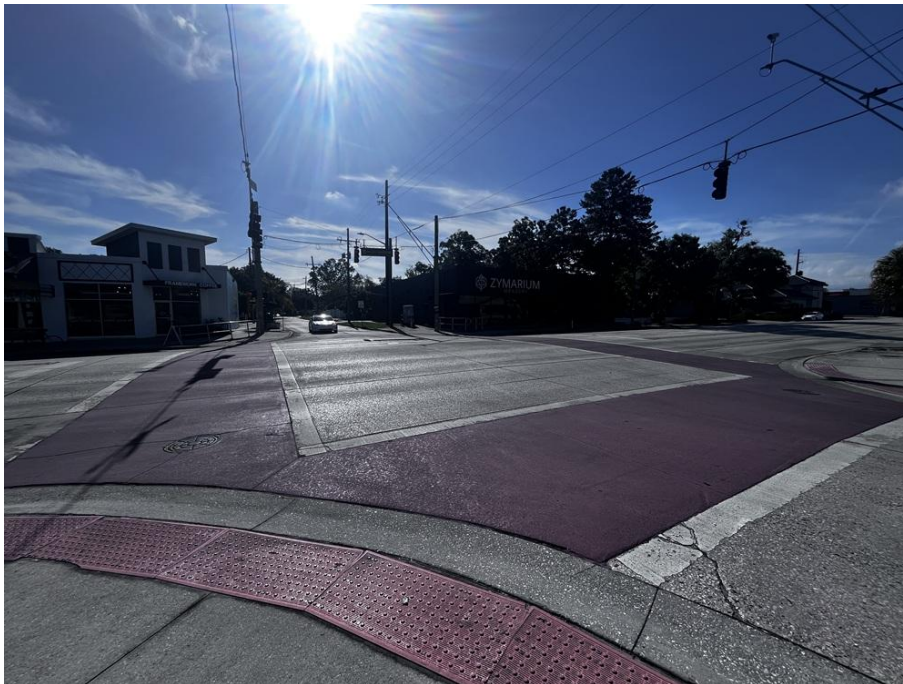
View east of Mills Ave and Lake Highland Dr Intersection
