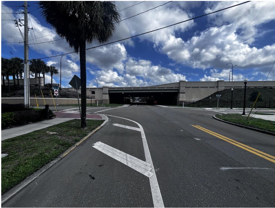
View south of SR 408 on Parramore Ave
