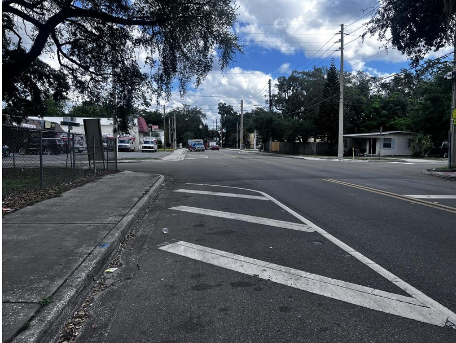
View north of Parramore Ave from south of Piedmont St at Gore St intersection
