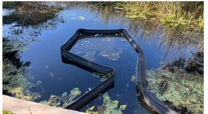
7 Trash accumulation in lake - Unsanitary or unsafe conditions.
