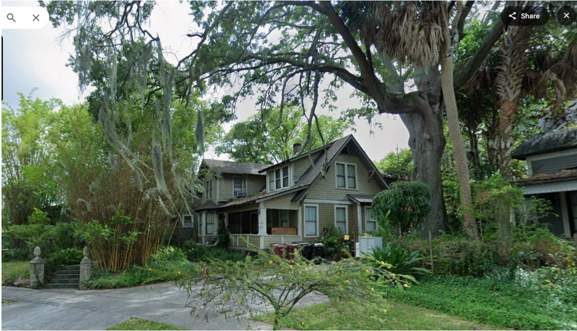
Original House that was demolished in 2023.
